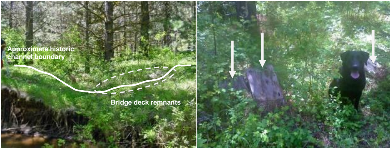
Figure 9. Inlet to historic channel (left). Arrows indicate bridge deck remnants (right).
