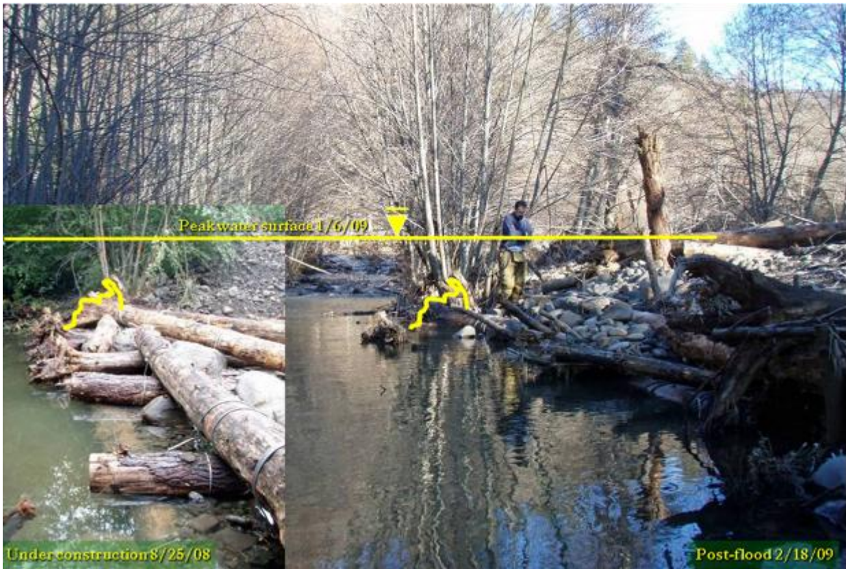
Figure 19. Element 4 during construction (inset) and post-flood.
